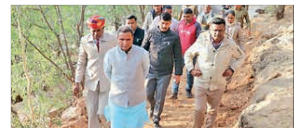
Dharmendra Rathore inspecting construction works being carried out to develop a tourist spot in Kazipura village near Foy Sagar Lake.
